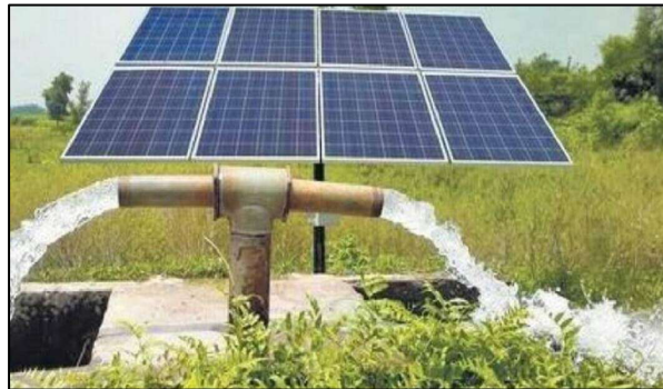
Figure 1 A solar Irrigation pump (source: Sarkariyojana.com)
